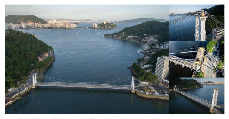
The São Vicente Suspension Bridge was erected in 1914 as part of the sanitation plan of the Santos and São Vicente area. Bridge condition in 2012 was deemed to be critical as some elements in trusses had disappeared and cable shown important corrosion and loss of cross section.
